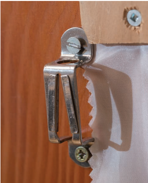
Marine cleat attached to the back of a framed artwork. Photograph by Kate Whitley © Te Papa
