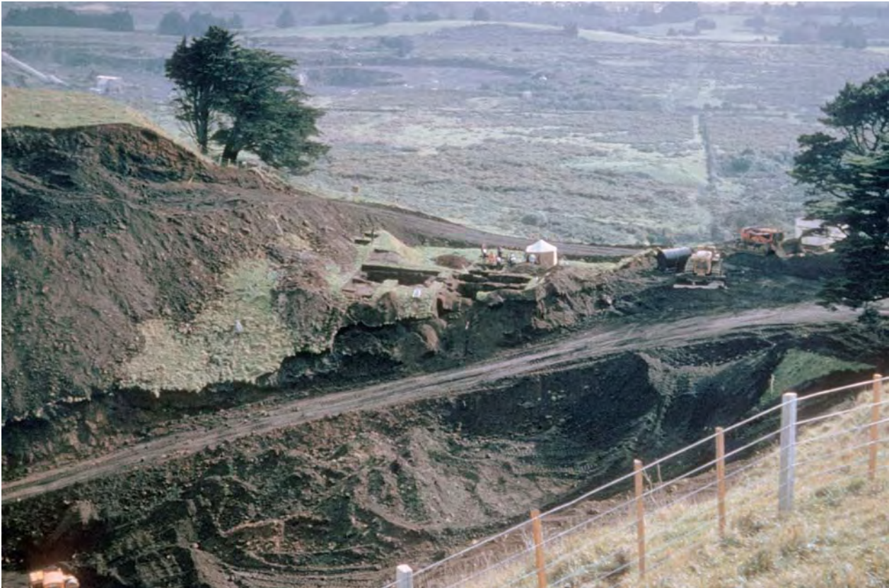
Fig. 13 Reservoir construction engulfs the excavations in Area A, June 1961 (photo: Bob Jolly).
