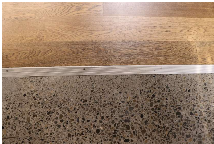
Image 6: Metal strip between wooden and concrete flooring.
