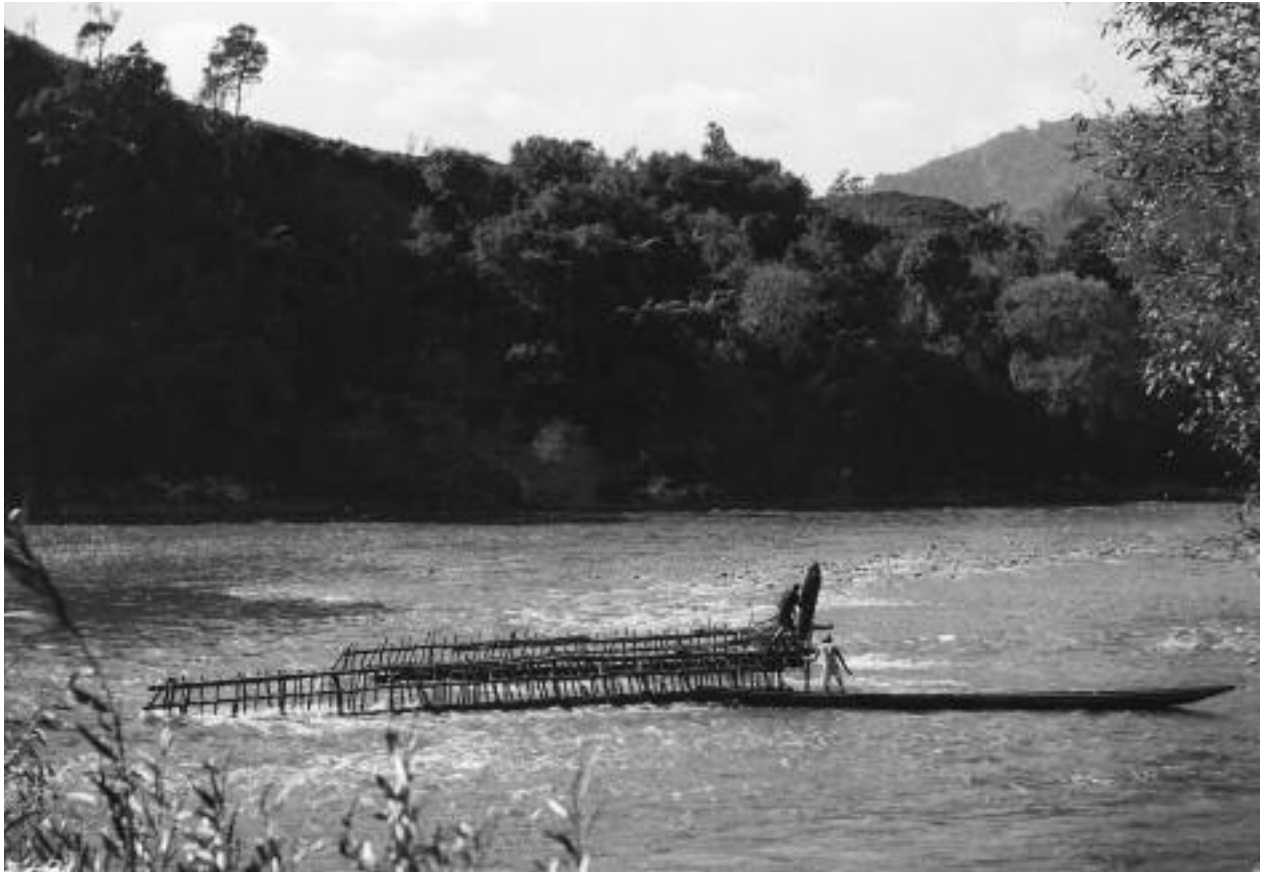
Fig. 4 Pā tuna eel weirs were designed to harvest tunaheke or migratory eels; the fence structures were up to 400 yd (370 m) in length and guided eels moving downstream into a funnel-shaped net (purangi). Eel-pots (hīnaki) attached to the net were emptied regularly from canoes. Whanganui River (photo: Te Papa, MA_B.000826, by James McDonald, 1921).
