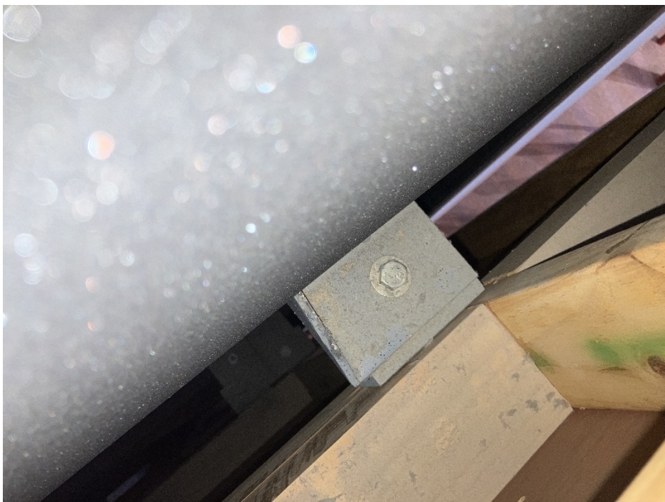
Image of Top Panel – one of the 3 fixings along the top of the artwork panel.
